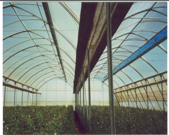
b) Inside a GH showing a thermal screen
