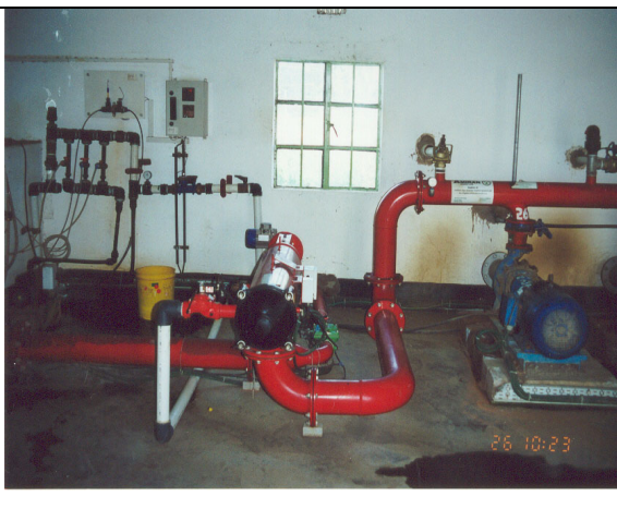
f) Pumping unit showing the filter
