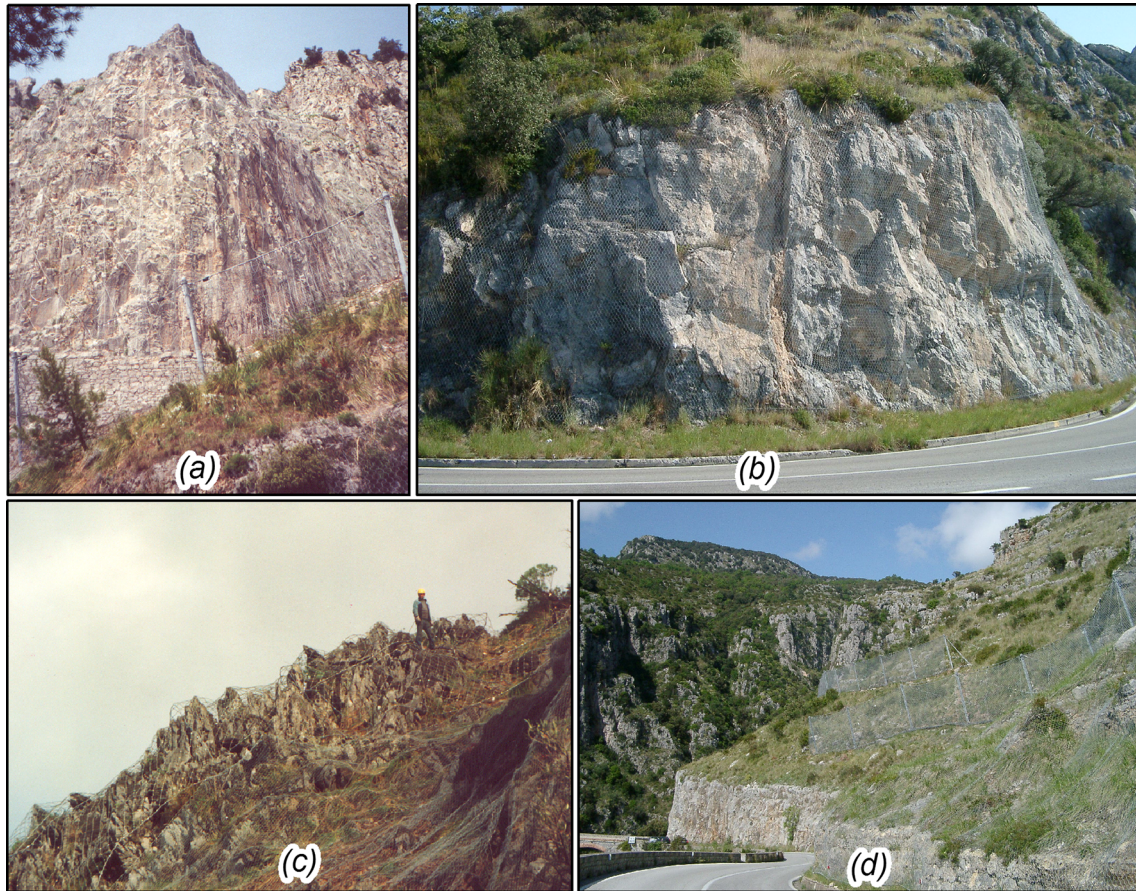
Fig. 6 Examples of defensive measures distributed along the SS18 in 2004: a surficial reinforcing revetment nets, b fixed drapery double twisted wire mesh, c surficial reinforcing panels, d rockfall catch fences
