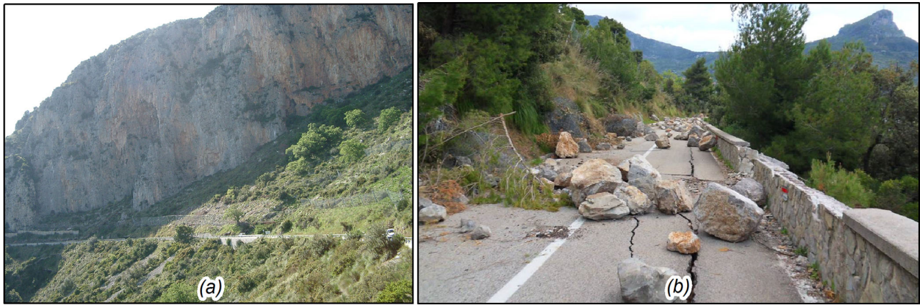
Fig. 2 Photos of steep and fractured rock slopes overhanging the SS18 coastal road (a) and rockfall on the road (b)
