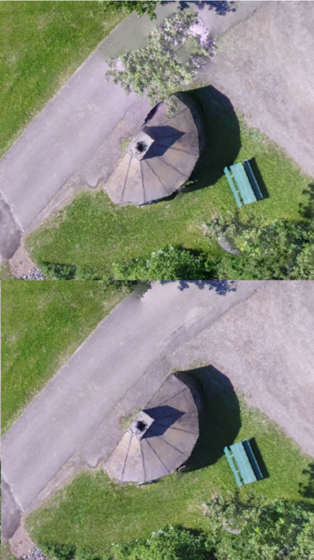
texturing-nadir-weight set to 0 (top) and 32 (bottom). Note the quality improvements near the edges of the building
