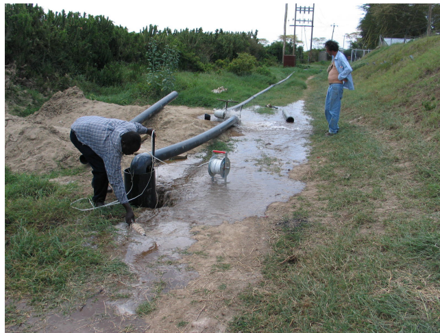
Few to mention problem during the injection test pipe
