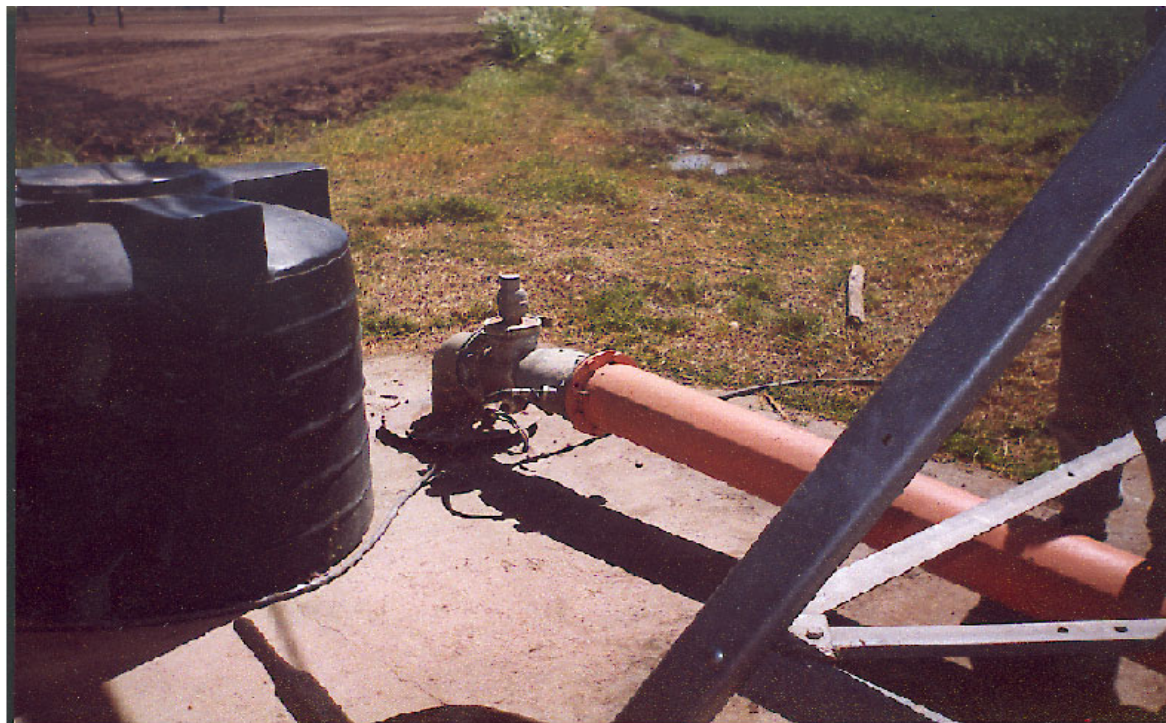
Plate 4: Borehole with Pump-intake fitted in Three Point farm.
