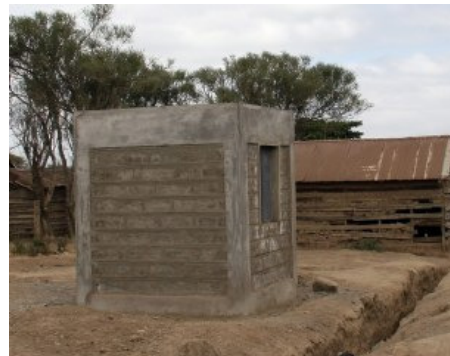
One of the water kiosks already in place in Karagita (2009)
