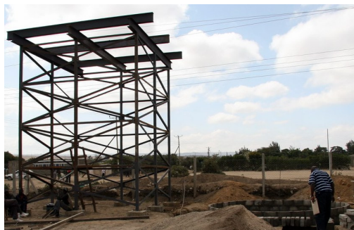
Support structure for soon-to-be installed raised water storage tank at the storage site in Karagita (2009)
