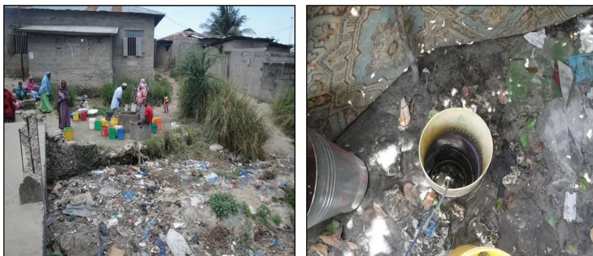
Picture 6-3 Unprotected communal borehole (left) and private borehole (right) in unhygienic places.
