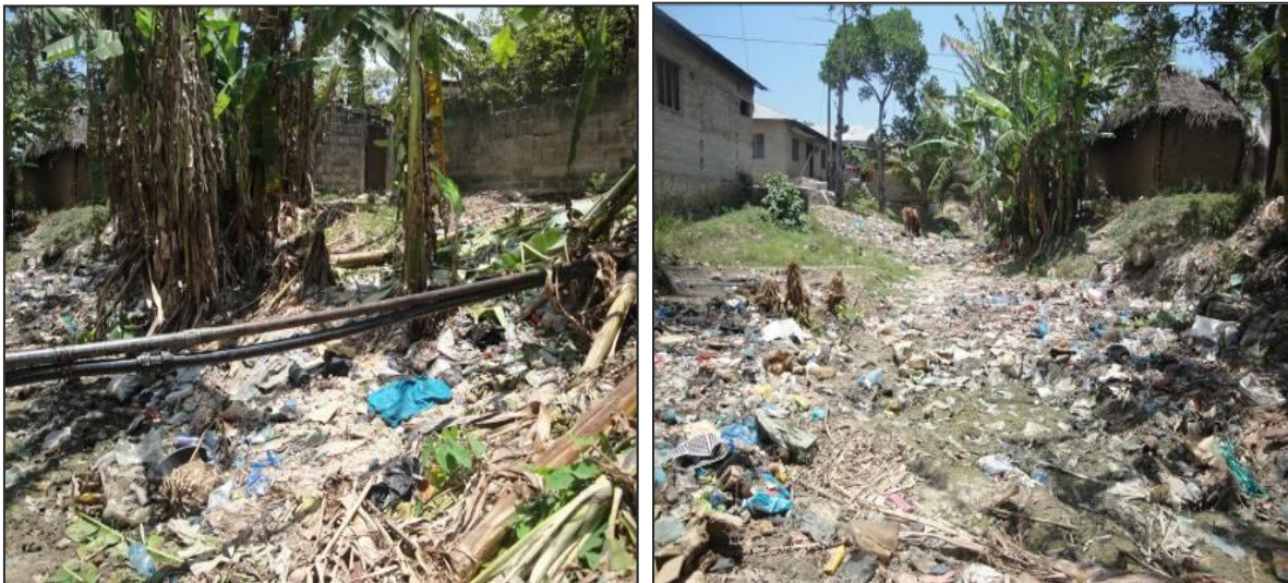
Picture 6-4 A storm water ditch-cum-dumping site showing loosely exposed water pipes traversing across the ditch and houses located very near the trench
