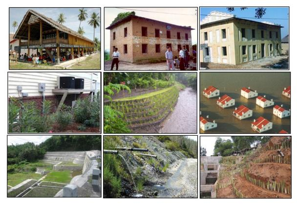
Figure 7.22: Examples of structural mitigation measures. Above: Raised community centre (tsunami hazard), and school retrofitting (earthquake hazard). Middle: raised electrical connection, gabions with vegetation for flood control and floating houses (flood hazard). Below: Retaining walls, slope drainage and biological engineering (landslide hazards)
