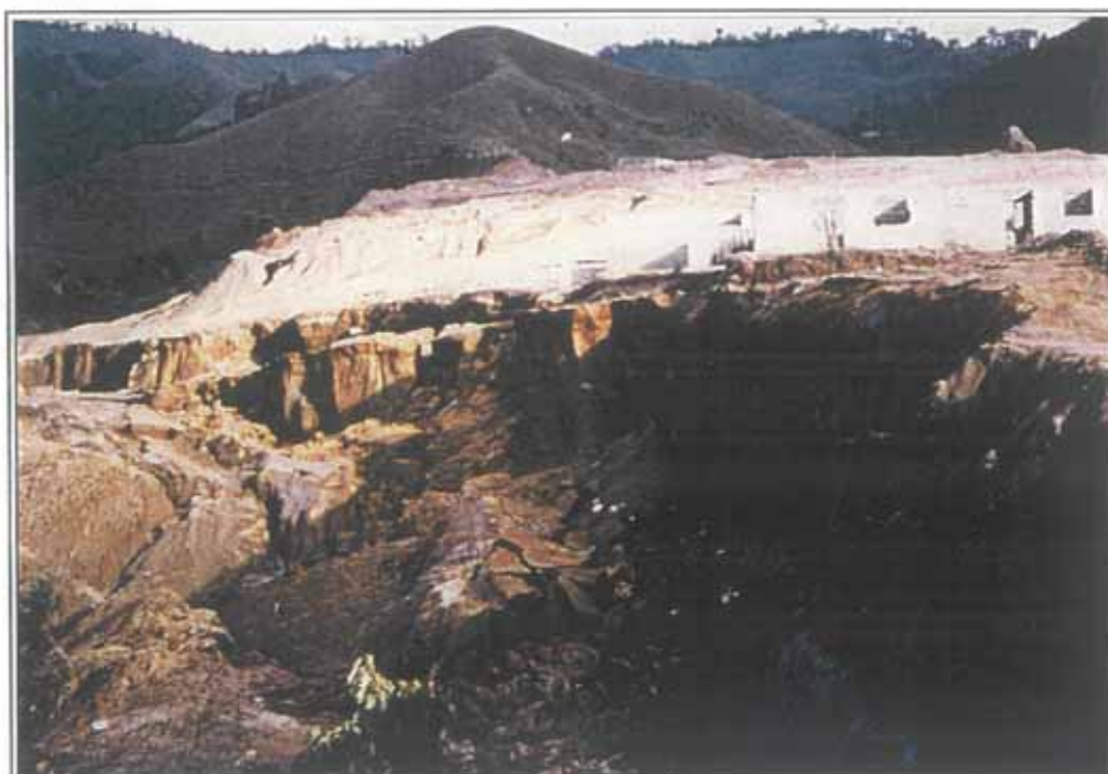
Figure 3.6: Seismic hazards in the Rio Chinchina catchment. Damage to newly constructed township in Manizales (Barrio Soferino) caused by a landslide triggered by the earthquake of 23 November 1979.
