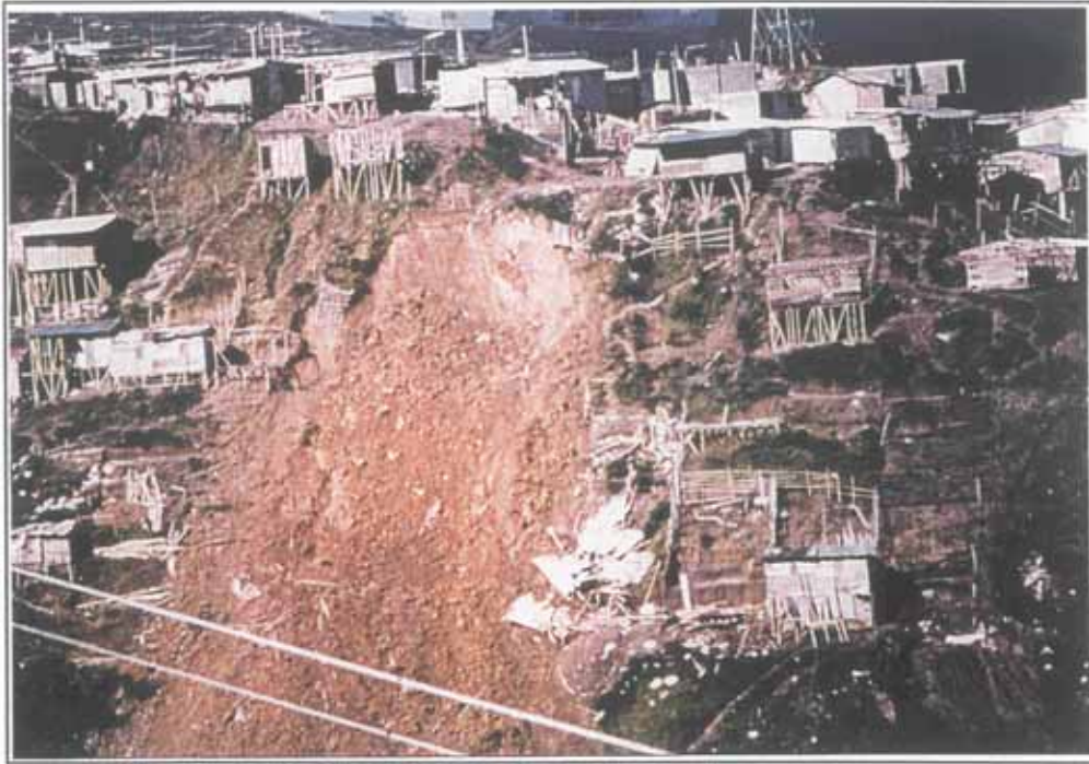
Figure 3.7: Landslide hazards in the Rio Chinchina catchment. Catastrophic rapid translational slide in a squatter area.
