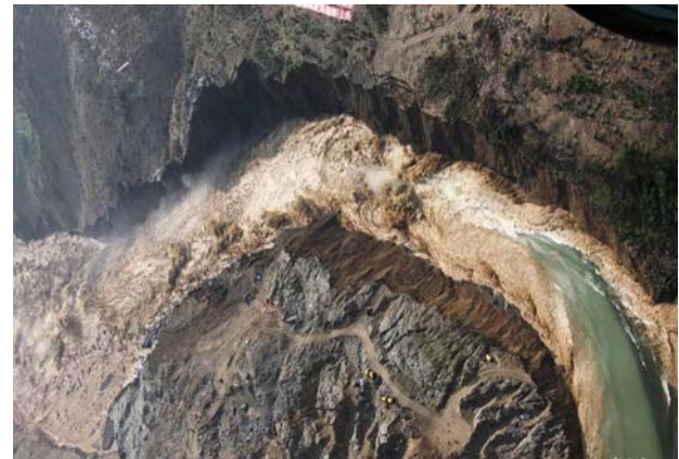
Fig. 13 Impounded water flowing through the artificial spillway. Taken at 11:00 (Beijing time) 10 June 2008 when the discharge reached its maximum (source: Liu 2008)
