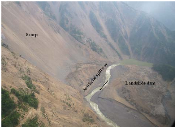
Fig. 12 Helicopter view of the artificial spillway in the Tangjiashan landslide dam
