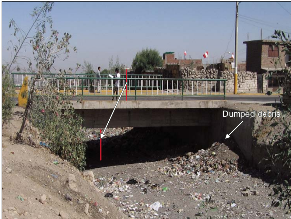
Figure 9. Huarangal pilot area: Infrastructure (roads and bridges). This bridge (Paucarpata–Mariano Melgar) along the Avenida Castilla is not only vulnerable to lahars because it is too low, but it could also increase hazard levels in surrounding areas by blocking the flow and creating overflow. Constant dumping of debris does not help either.
