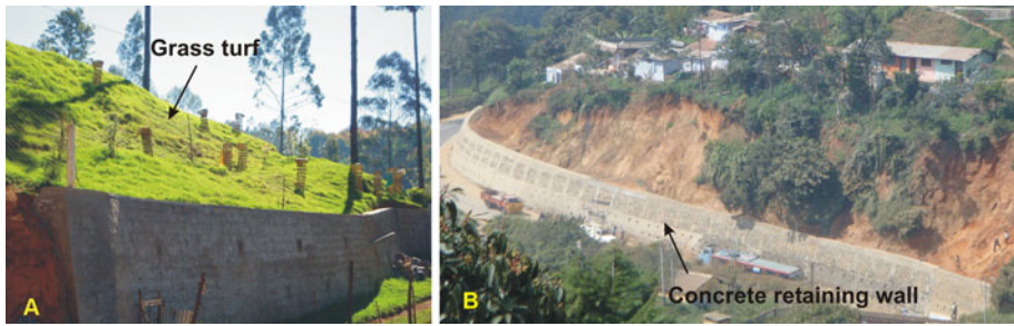
Fig. 7 Slope stabilization measures: a grass turf combined with retaining wall and b concrete retaining wall
