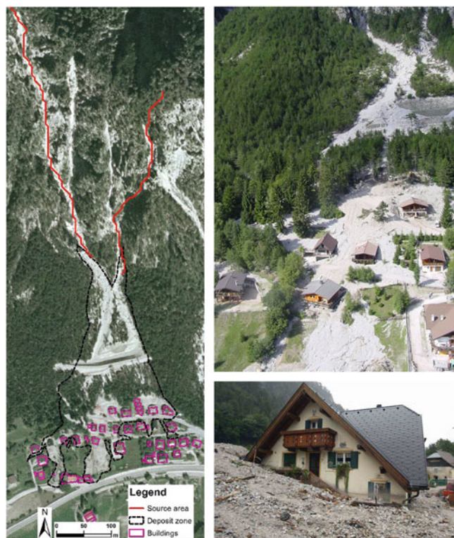
Fig. 1 (Left) The Abitato Cucco 2003 debris flow from the initiation to the deposit zone and (right) the breach of the barrier which damaged several houses
