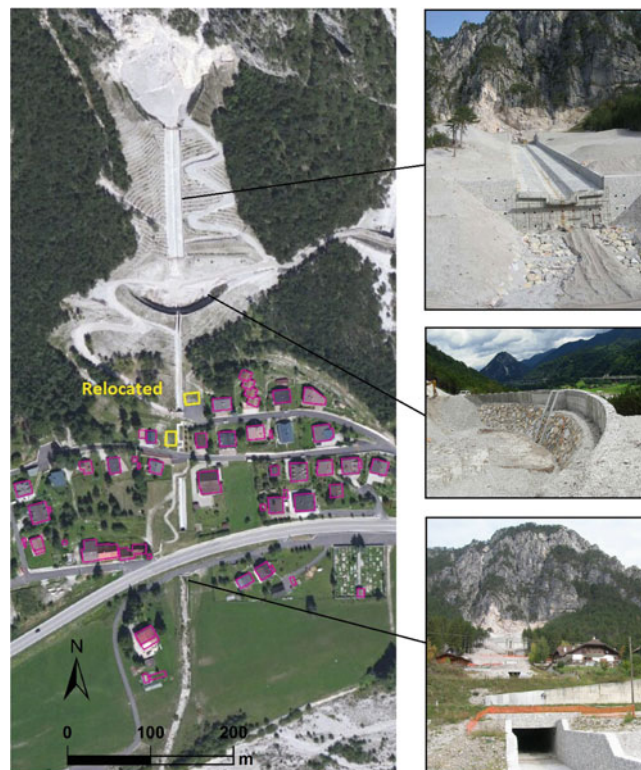
Fig. 2 The mitigation measures constructed at the Abitato Cucco basin following the 2003 event, including the two houses that were relocated
