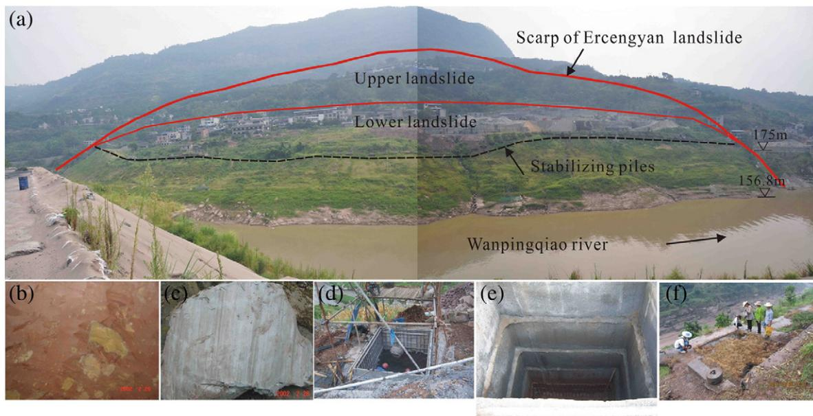
**Fig. 2.** (a) Photo of Ercengyan landslide and stabilizing piles; (b) Silty clay with gravels in the sliding soil (photo taken in 2002); (c) Striations on the slip surface from the shaft (2002); (d) Cast-in-place reinforced concrete piles (2006); (e) Reinforced concrete retaining wall inside pilehole (2006); (f) Top of a 3 × 4.5 m rectangular pile (2007).
