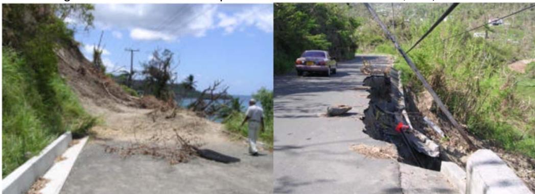
*Figure 4-8: Landslides affecting the road network caused by Hurricane Ivan in 2004. Left: Landslide at St. Paul's; Right: Landslide at Grand Etang and Westerhaul.*
