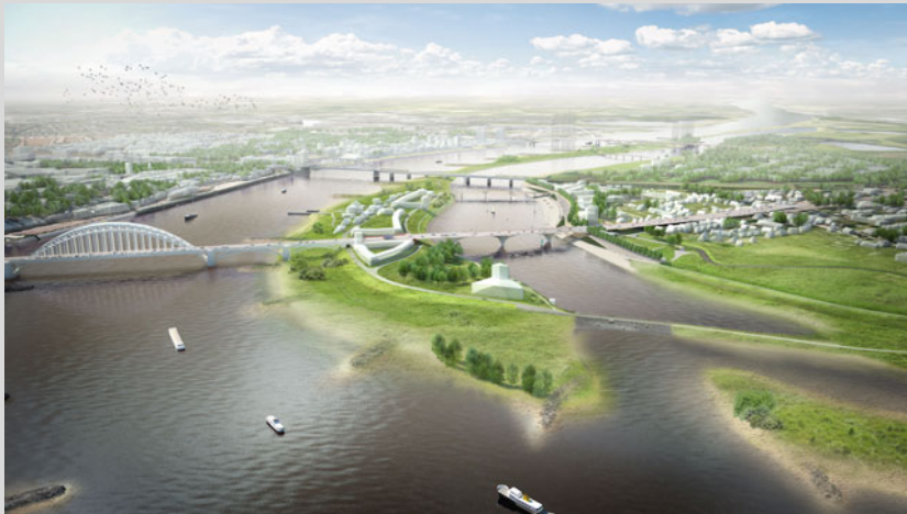
Fig. 7.1 3D-impression (downstream view) of the expected results of the Room for the River project at Nijmegen. River bend in Waal river ( left side ) and construction of an ancillary river channel ( right sight ) create a new island for recreation and re-establishing natural values (Image: Room for the Waal Nijmegen, ( www.ruimtevoordewaal.nl ), used with permission).
