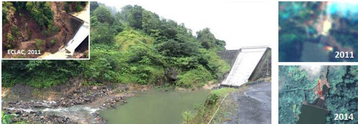
Figure 4-12: Landslides near the Roseau Dam. Multiple events in 2010 seriously affected the water quality of the reservoir and a large landslide occurred to the east of the dam (see inset photo from ECLAC 2011). The remains of this landslide are still clearly visible. The direction of the photo is indicated by a red arrow on the satellite image of 2014. Compared with the 2011 image it is evident how much more detail can be observed.
