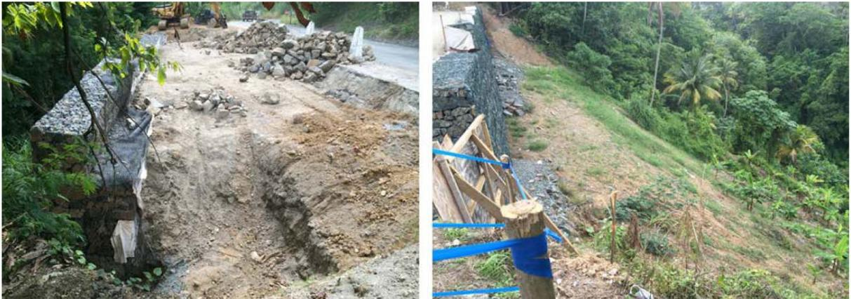
Figure 4-15: Landslide stabilisation works along the Vieux Fort-Castries road at Thomazo
