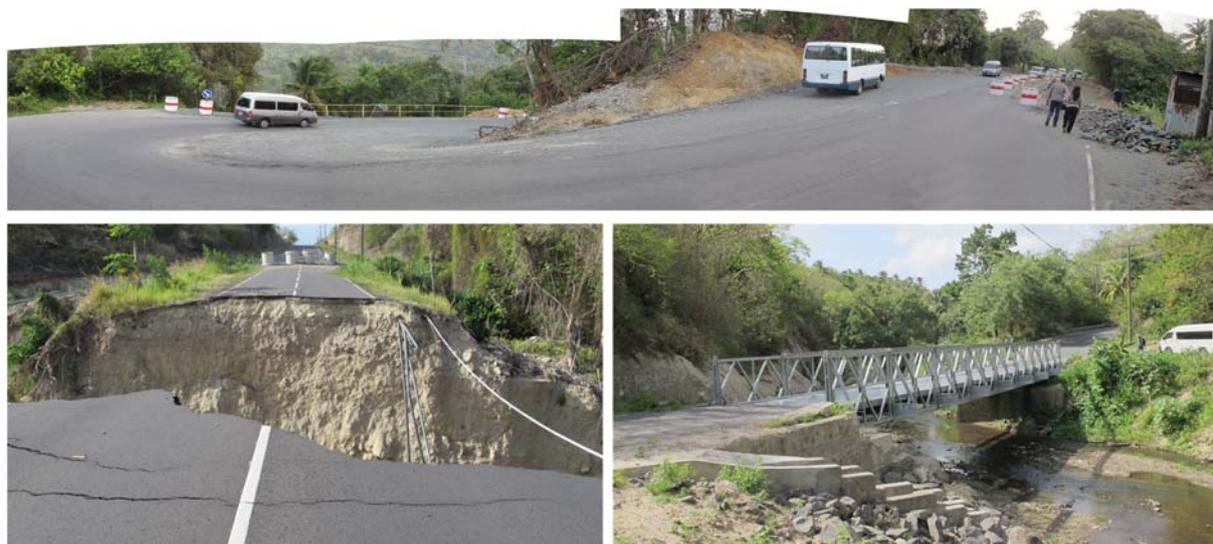
Figure 3-3: Some of the damaged areas during the 2013 Christmas Eve event. Above: landslides along the road to Dennery. Lower Left: culvert failure leading to road collapse and two casualties along Micoud Highway in the Southeast. Lower right: Bailey bridge due to bridge washout at Sapphire (Southwest).
