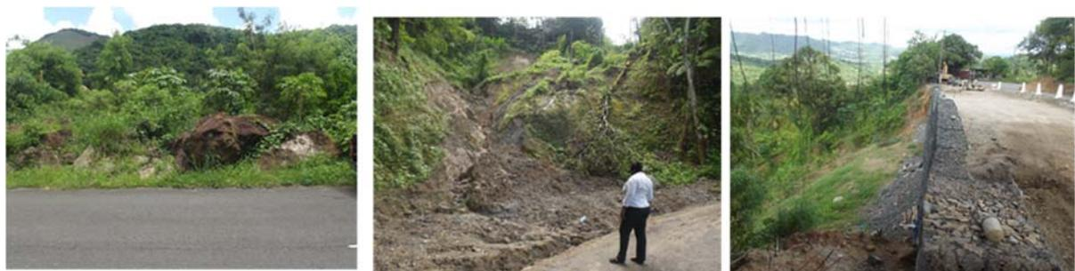
*Figure 3.2: Landslides along the major roads of Saint Lucia, resulting from Hurricane Tomas that were still visible in 2014*
